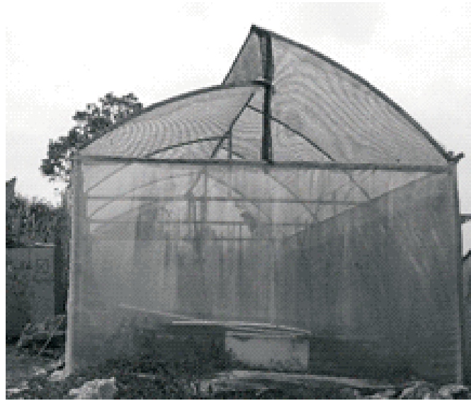
FIGURE 3: Single ridged vent gable roof greenhouse, Clarendon
